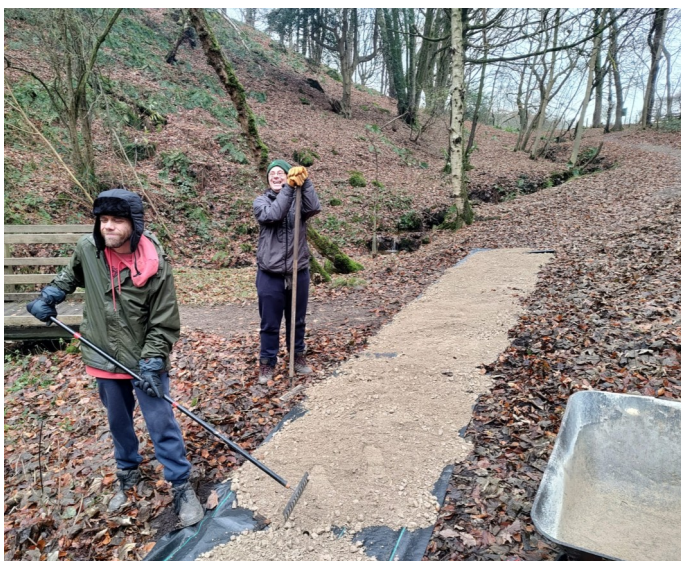
Our volunteers hard at work laying the new path
